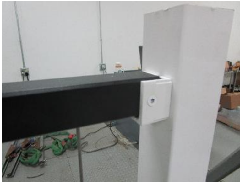
Photo No. 7 Cast Aluminum Bracket for Level Top Rail
